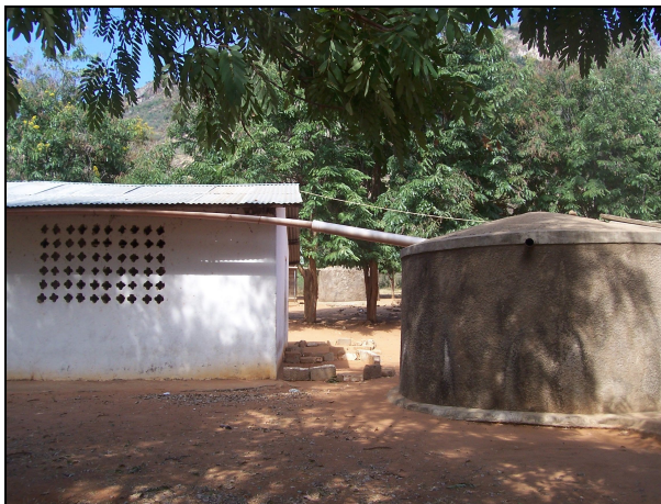
Figura 5.17: "roof catchment" della Hawecha Primary School
